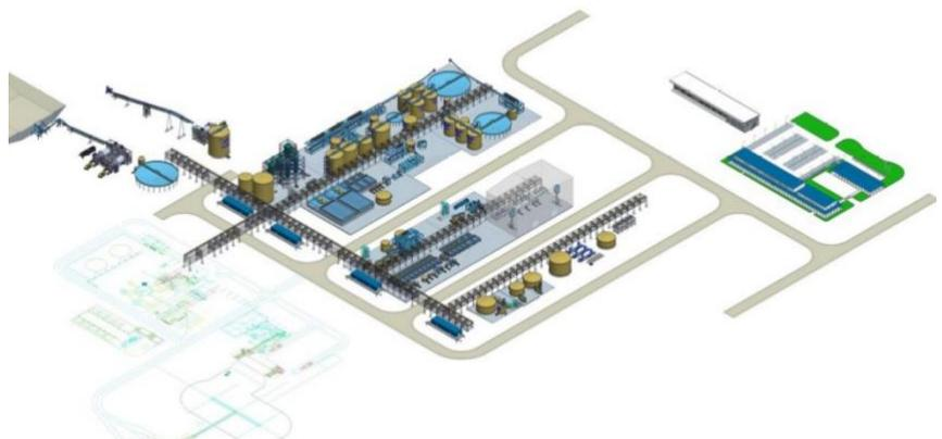
Ore from Sconi was processed through the High Pressure Acid Leach (HPAL) circuit at the demonstration plant, with the resulting leach liquor then taken through scandium solvent extraction, scandium precipitation and calcination, iron removal and mixed sulphide precipitation (MSP). The resulting MSP was then fed through the refinery circuit, which includes pressure oxidation followed by impurity removal, cobalt and nickel solvent extraction and crystallisation steps.
